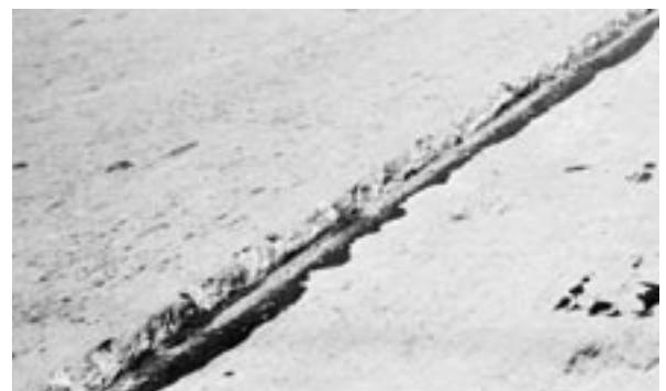
▲ Faulted longitudinal joint.
