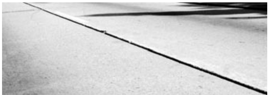
▲ Faulted longitudinal joint.
