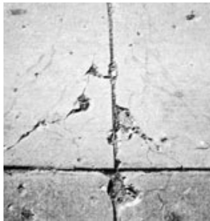
Corner cracking with broken concrete pieces.
