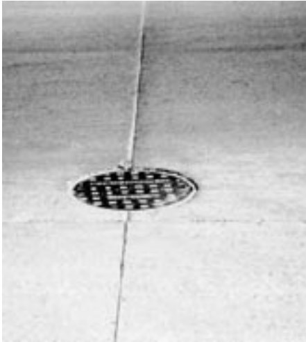
▶ Severe spalling of a transverse joint.
