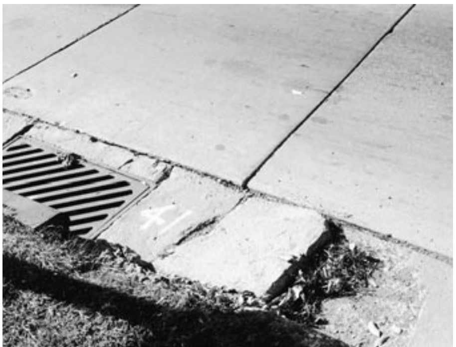
Extensive curb deterioration. Freeze-thaw damage to curb adjacent to inlet, and gutter is displaced. New curb and gutter are needed. ►
