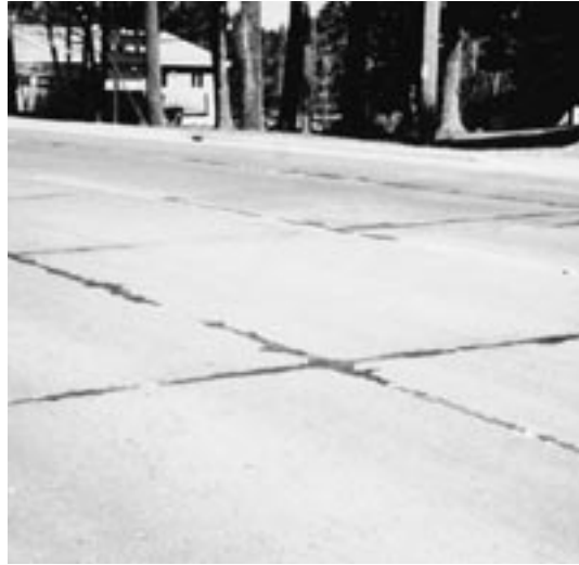
◀ All joints show some deterioration and spalling.
