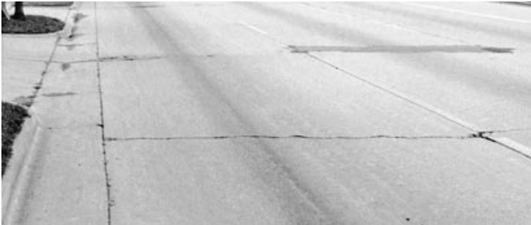
◀ All joints show some deterioration and spalling.
