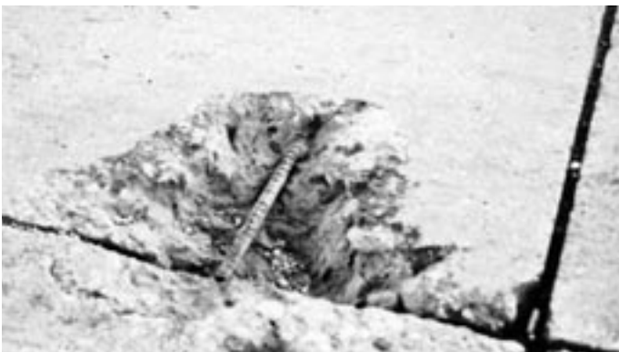
Reinforcing bar exposed. Shallow concrete cover caused large spall to develop around it. ▼
