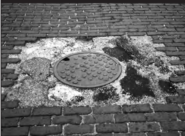
Manhole repairs leaving surface in very poor condition.
