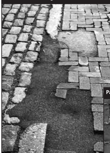
Patches for missing bricks and blocks.
