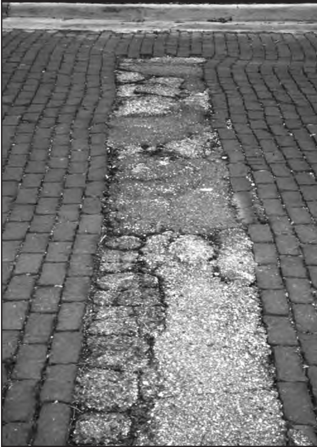
Manhole repairs leaving surface in very poor condition.
